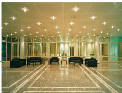
Molded case circuit breaker for line, personnel, and fire protection inside the building
